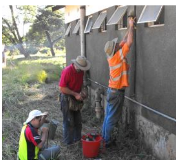
Craig, John and Peter repairing plumbing at Fiwale Hill
